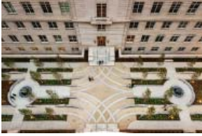
Image 2 The 21,000 square foot courtyard has a north- south axis between massive granite steps and two granite fountains at the ends of its east-west axes. A symmetrical medallion of concrete paving in a field of decomposed granite sets up the circulation pattern.
