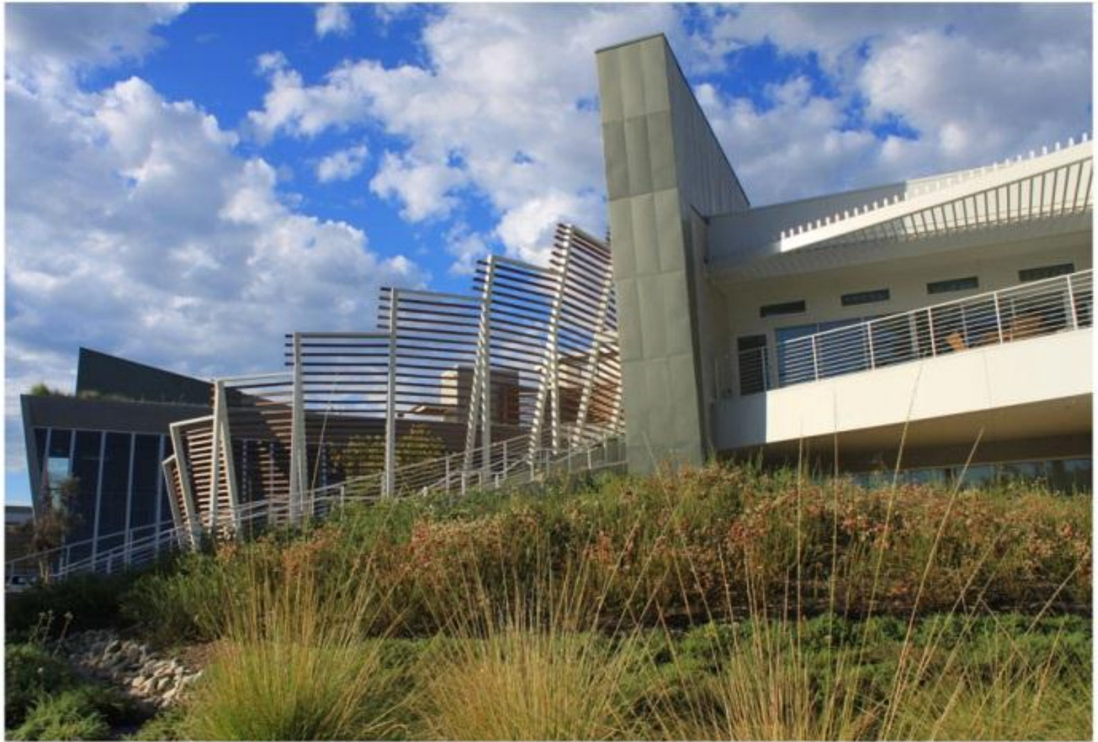
The excavated soil from the infiltration basin, cistern and rain garden was kept on site and used to create a Chaparral Hillside around the building's north wing.
