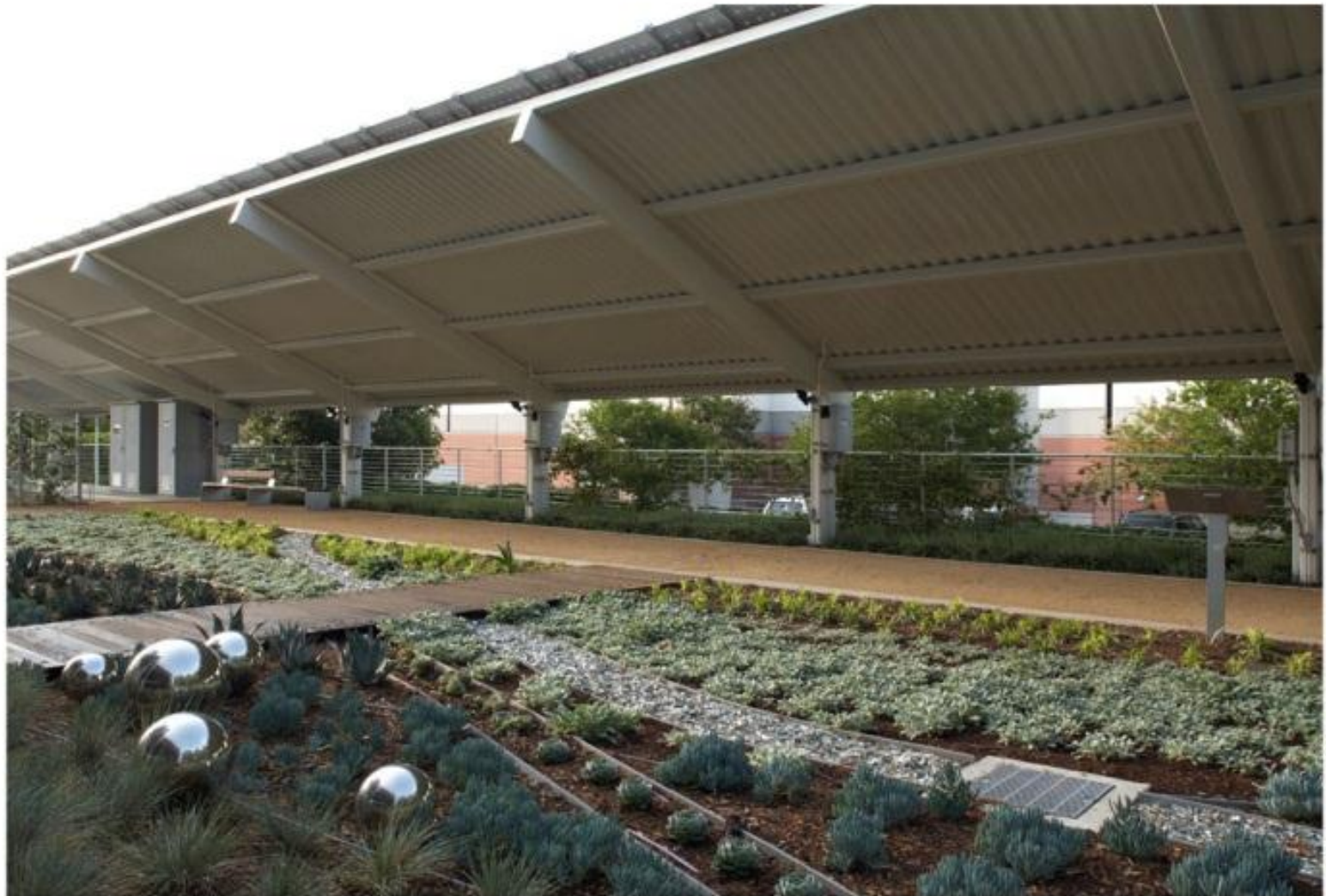
The "Water-Less" Garden lies over the cistern and infiltration basin. A shade structure supports photovoltaic panels. Drought-tolerant succulents and plants available at the local garden center demonstrate efficient garden materials for sun and shade.
