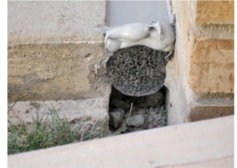
Backer rod with fresh mastic seal on top
