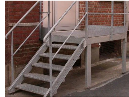
Industrial site with open riser stair
